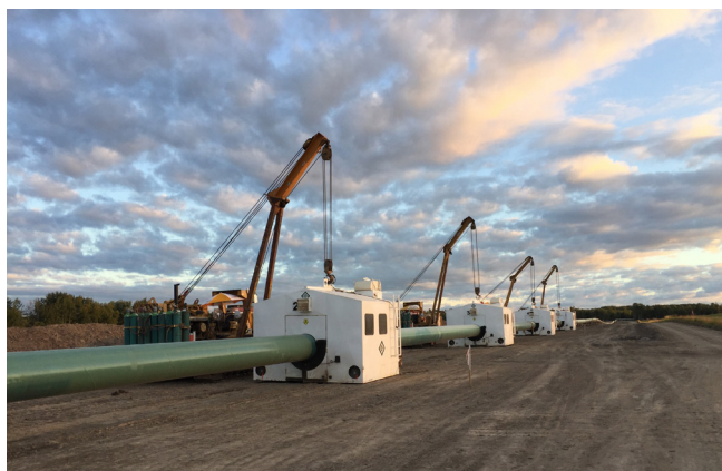
Figure 5. Welding on the right-of-way.
