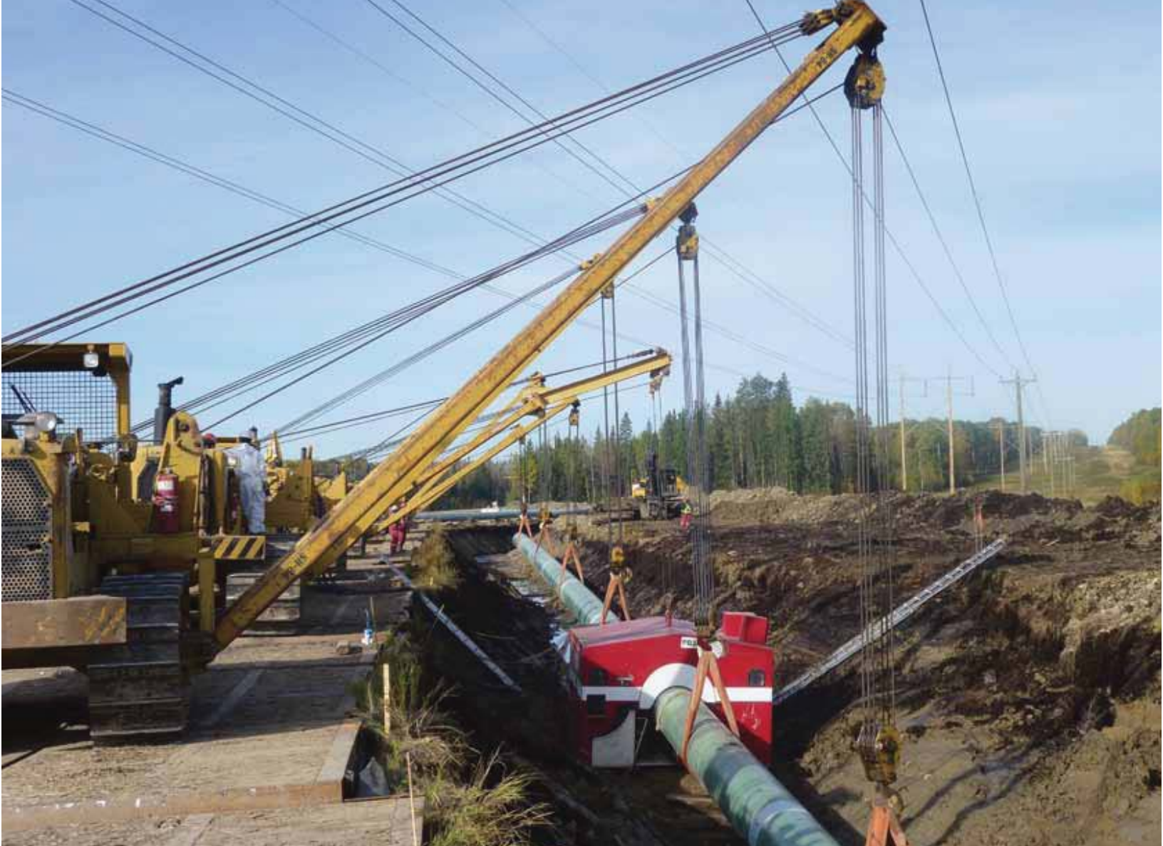
Figure 10 – A shack being placed for execution of a mechanized FCAW-G tie-in weld.
