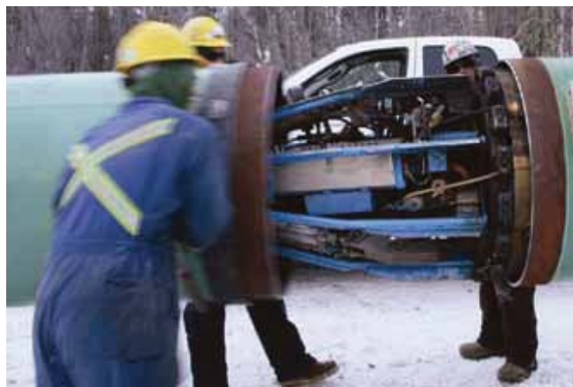
Figure 5 – Fitup being set between two pipes.
