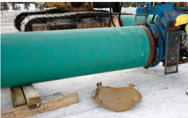
Figure 9 – End preparation machine bevelling a pipe end.
