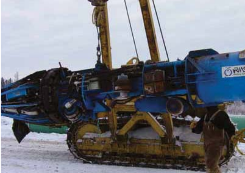
Figure 2 – An internal welding machine (IWM) being moved.
